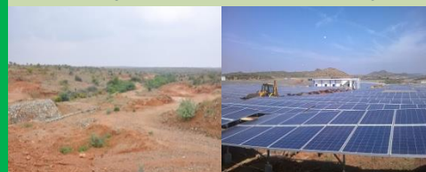
Transformation from barren land to 250 MW project in 1 year time
