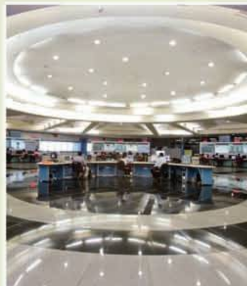
A View of NTPC Sipat Control Room
