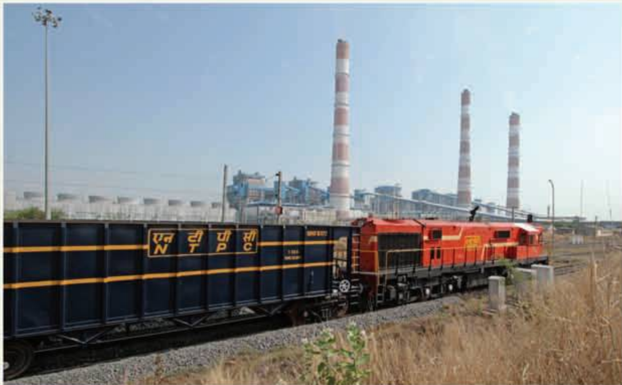
Coal transportation through MGR at NTPC Power Station
