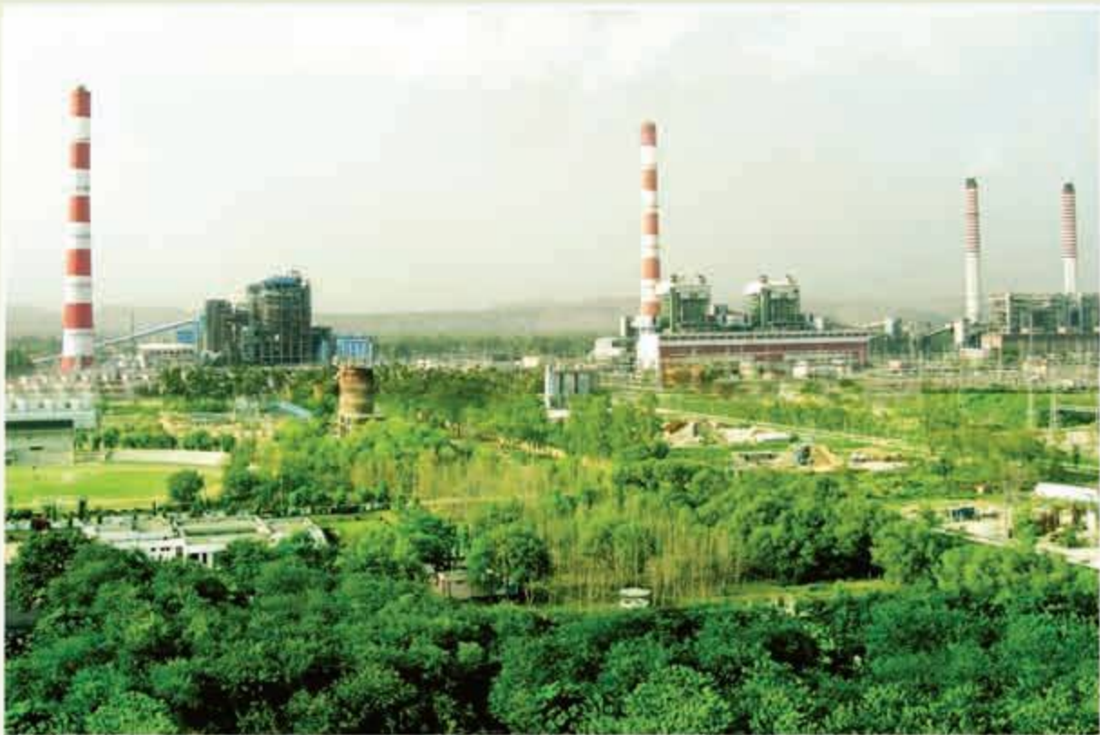
NTPC Vindhyachal - The largest power station of the country
