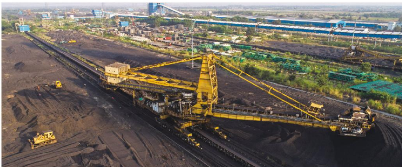
View of CHP, NTPC Talcher Kaniha
