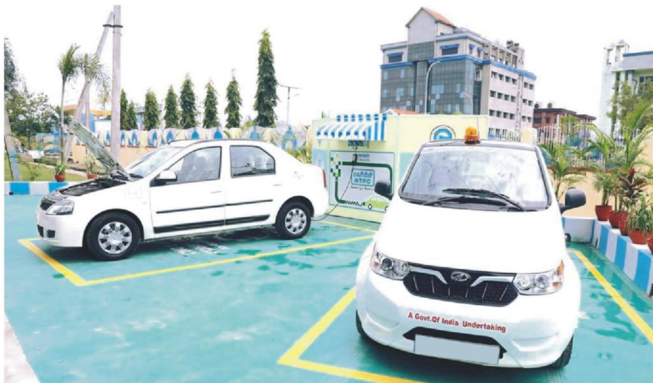
EV Charging Station at NTPC, Simhadri
