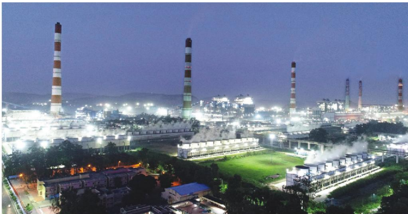
LED Illumination at NTPC, Vindhyachal
