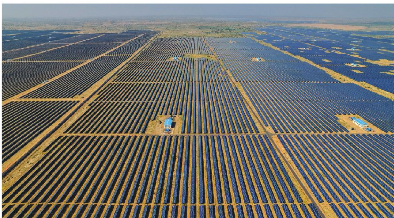
NTPC Bhadla Solar PV Plant
