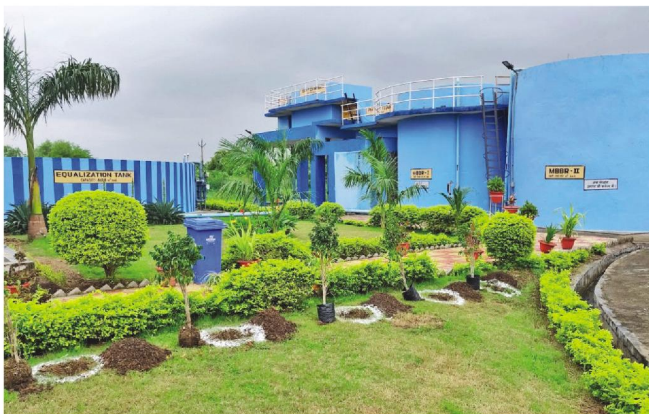
Sewage Treatment Plant (STP), NTPC Mouda
