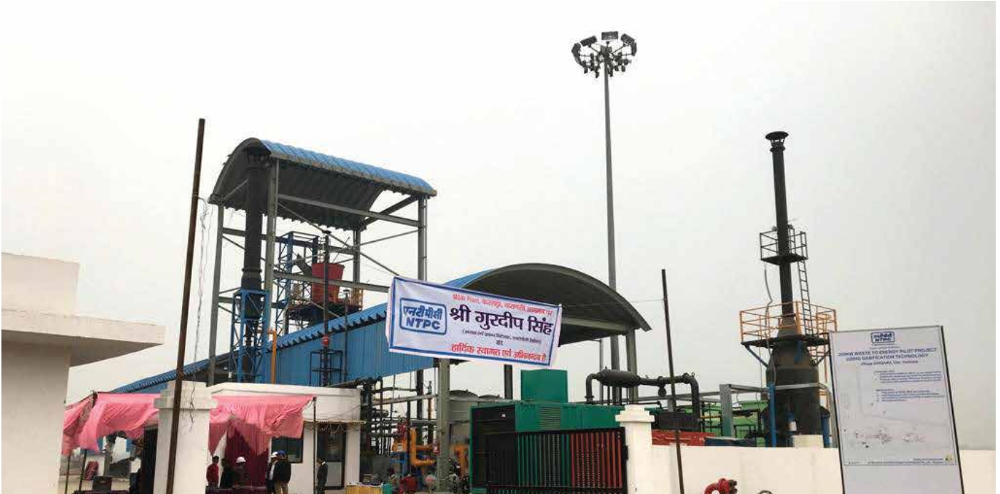
Waste to Energy Plant, Varanasi
